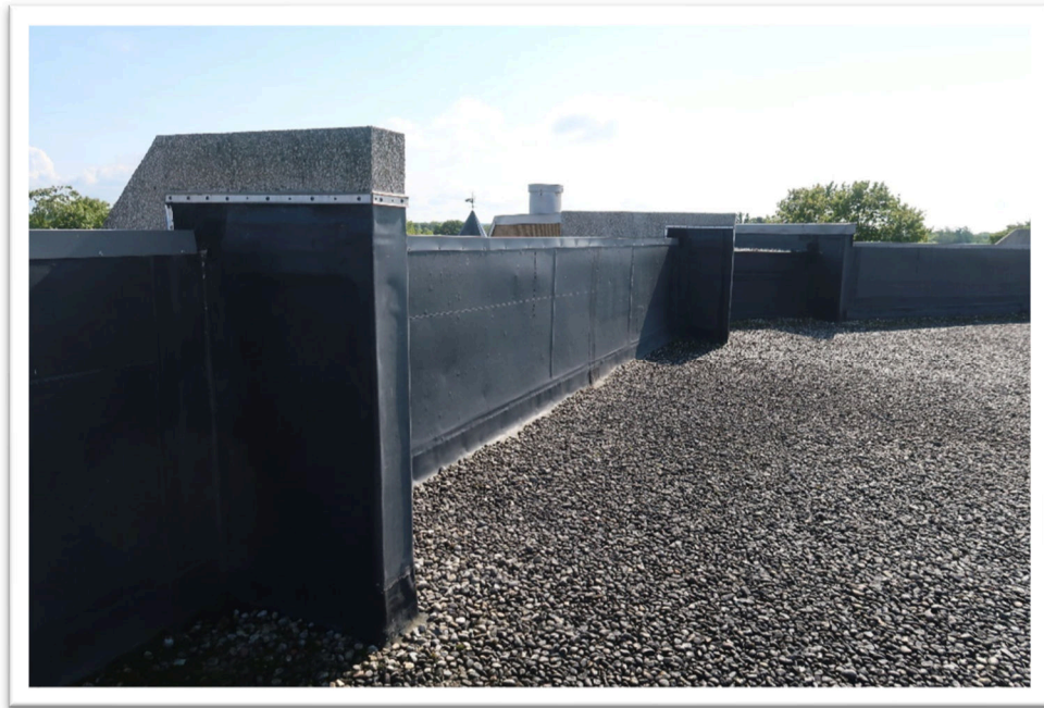
Photograph 11: Typical view of EPDM roof with stone ballast
